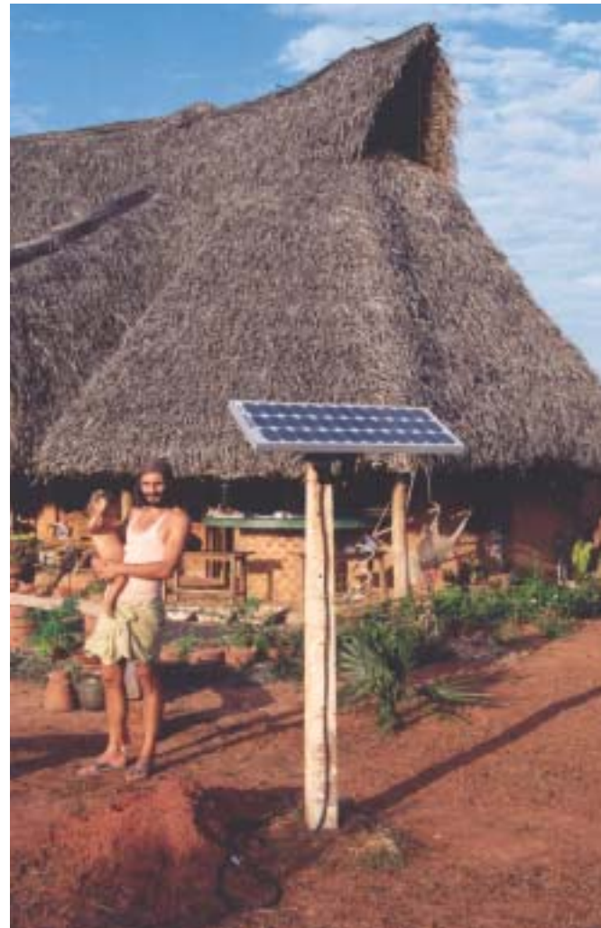
A small Solar Home System (SHS) in Auroville
